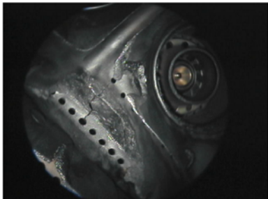
Figure 2-42. Trumpet Area Missing Material
