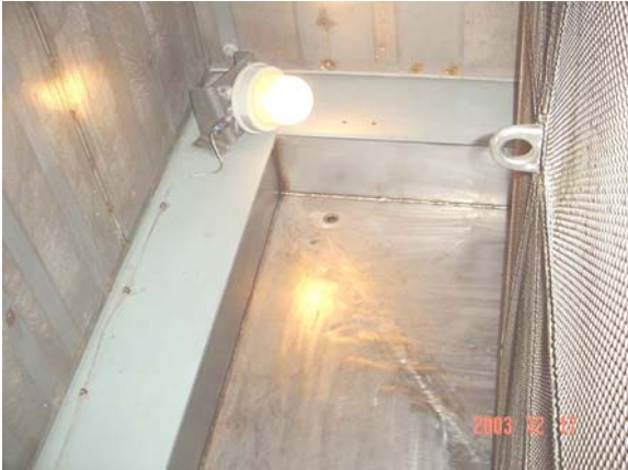
Figure 2-75. Clean Inlet Plenum
